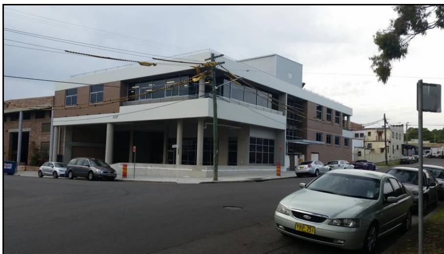
Photograph 1: The existing two storey building as viewed from the corner of Spencer Street and Regatta Road. The building's appearance is that of a commercial building, with two (2) floor levels and two (2) basement parking levels.
