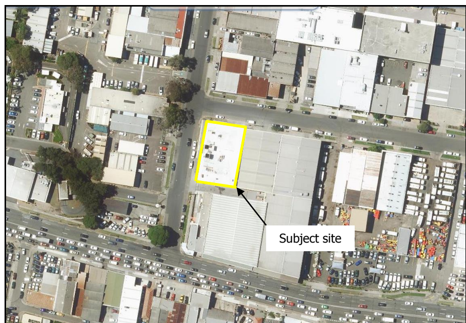
Figure 2: Aerial Photo of Subject Site (No.25-27 Spencer Street, Five Dock) Source: SIX Maps, NSW Government 2015
